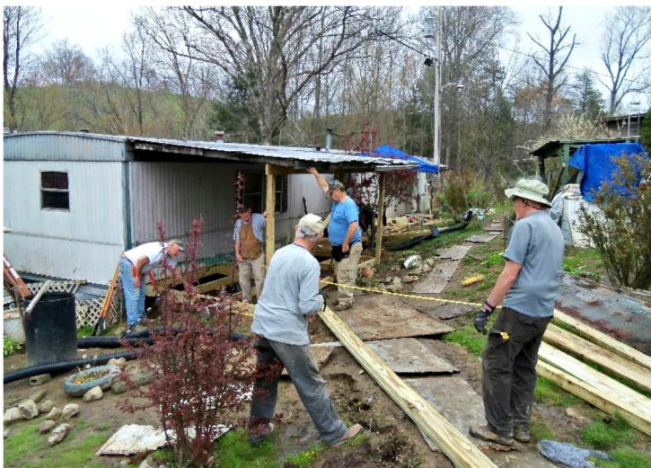
Laying the ramp from the deck to the driveway.
