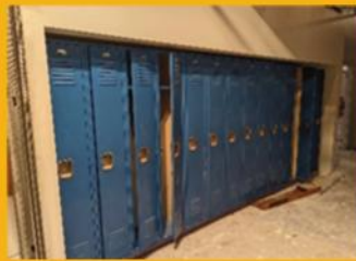
Start of Locker Installation
