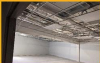
Grid Work in Classrooms
