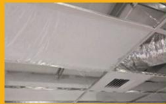
Vent & LED Panel Installation
