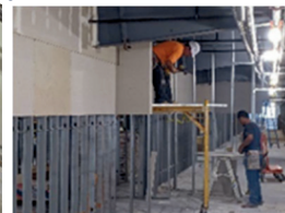
Hallway View of Classrooms
