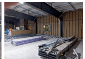
Inside view of ~20% of Chapel
