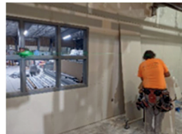
View Hallway from Classroom
