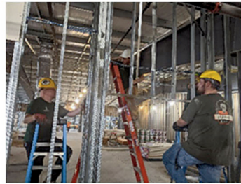
Pulling Electrical Cables
