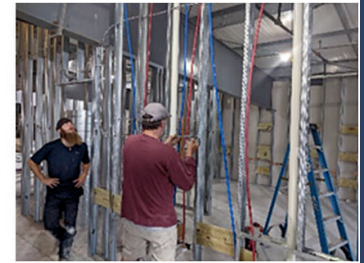
Installing Hot & Cold Water Lines
