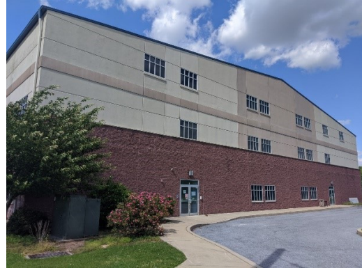
Exterior Surfacing & Resealing
