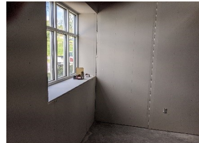
Admin offices drywall
