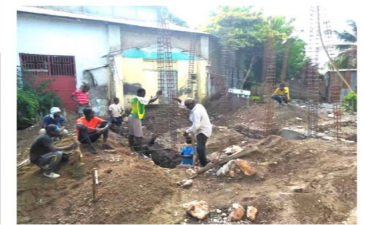
RECTORY - IN PROGRESS
